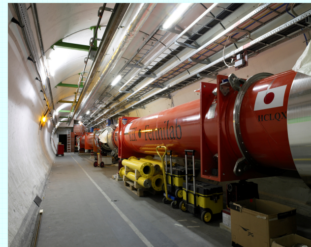
Installation in progress in LHC tunnel
